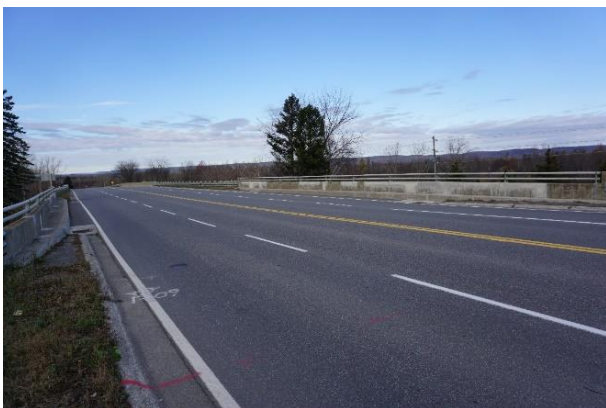
Figure 6: Typical condition of County Road 17 Underpass
