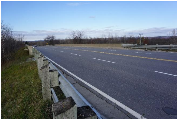
Figure 4: Typical condition of CNR Overhead
