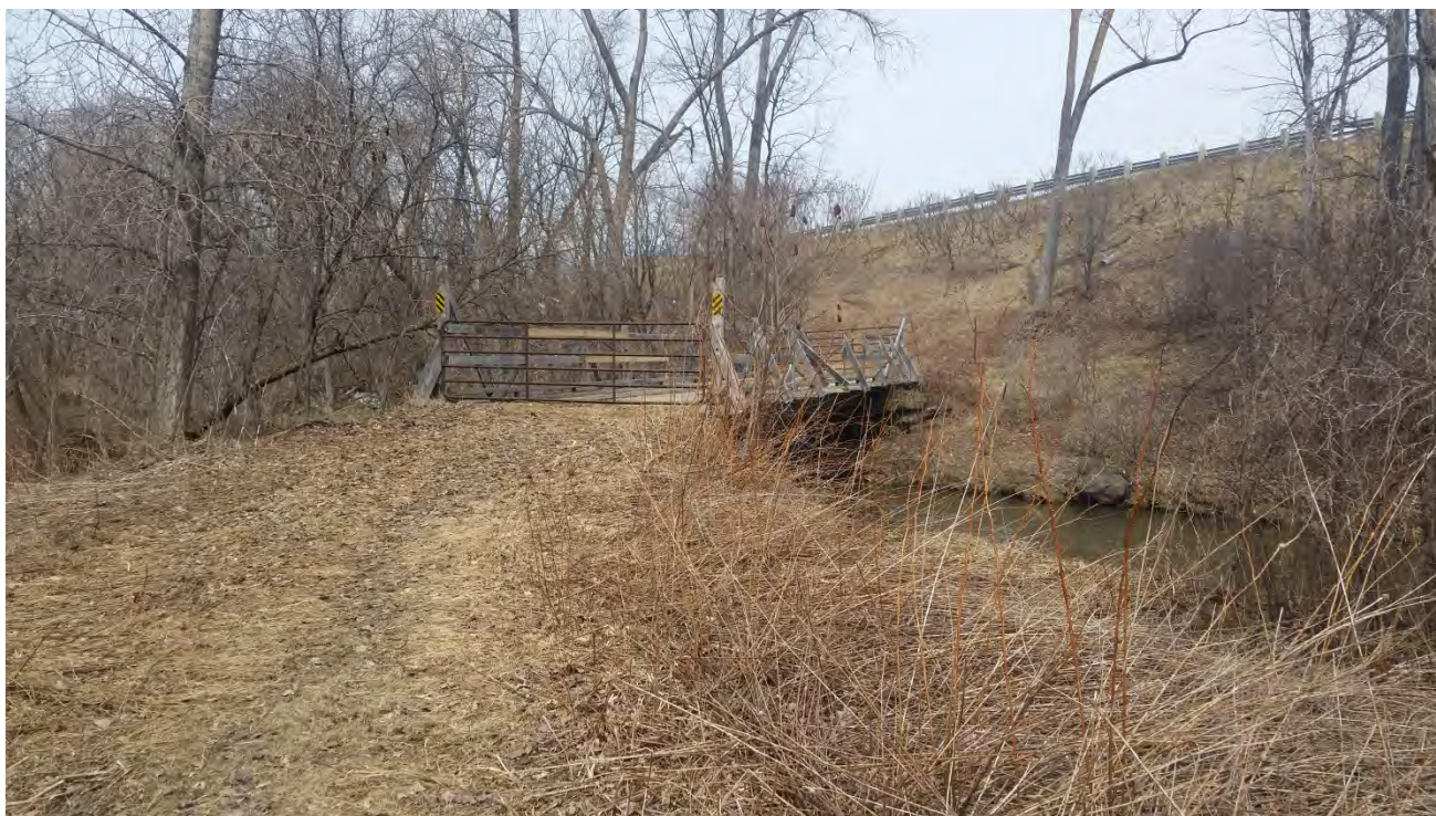
Image 21: Footbridge in south west quadrant facing north west.
