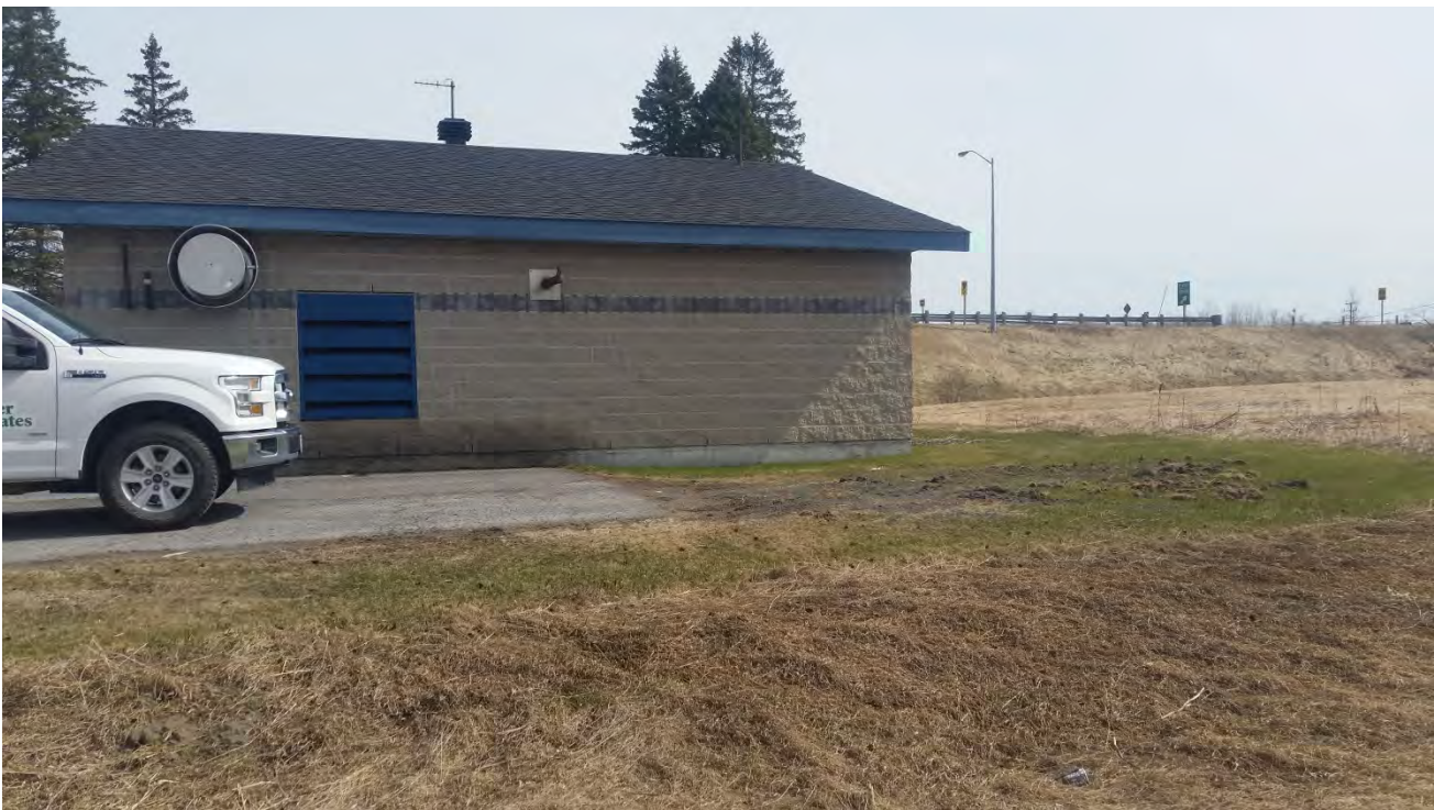
Image 2: Grey Stone building in southeast quadrant facing north.
